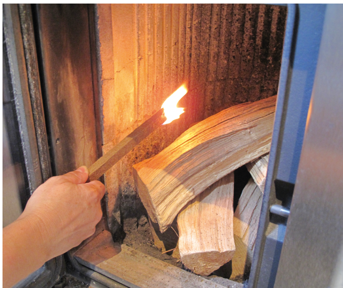
Check if there is sufficient negative chimney pressure ("draught test")
